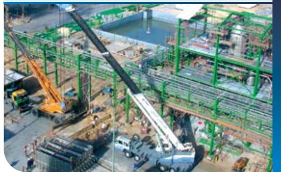
Pipe Rack / Equipment Foundations
